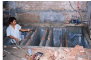
Baffled septic tank with anaerobic filter (BASTAF) Scheme and Construction
